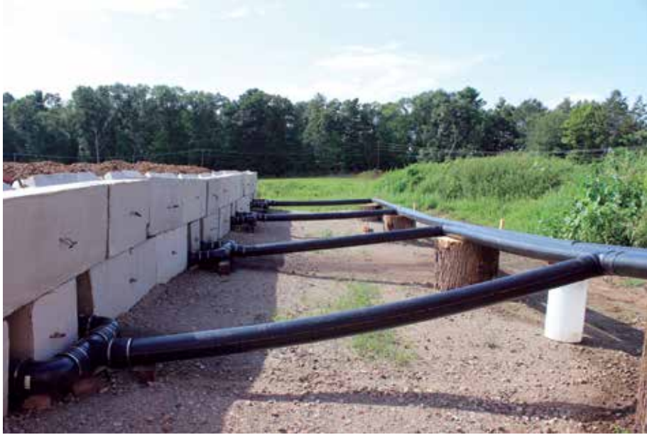
Aeration pipes that feed hot air from the compost windrows to the Hotskid.
