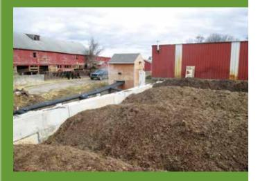
Four batches (110+ cubic yards each) of manure compost loaded into aeration bays at Collins Powder Hill Farm. Hot vapor is pulled to Hot Skid 250R unit inside shed for energy capture while accelerating the composting process. PHOTO CREDIT BRIAN JEROSE
